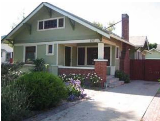
1921 Bungalow House in the Historic District of Anaheim
